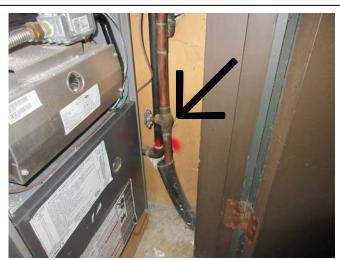
The house original supply pipes is copper. The life expectancy of copper piping is dependent on water condition, it may fail within 20 years. However the copper life expectancy is 40-50 years. The main water shut off valve is located in the furnace room of the house.
