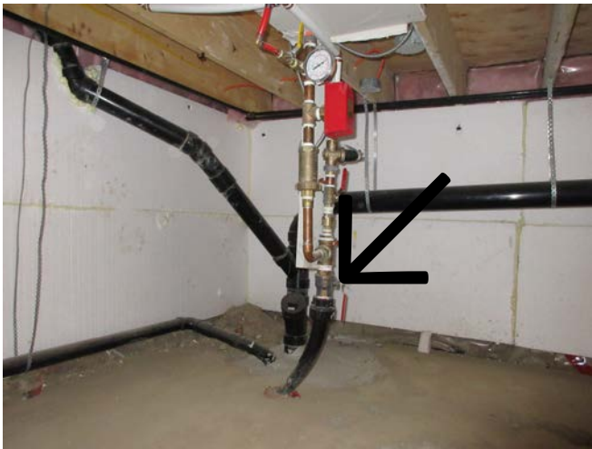
The main water shut off valve is located in the crawl space of the house.
