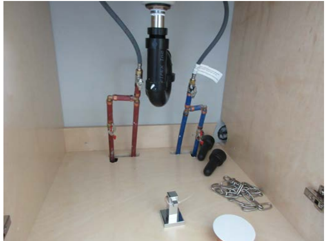
The house original supply pipes is PEX. The life expectancy of PEX piping is 40-50 years.
