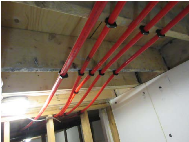
The house original supply pipes is PEX. The life expectancy of PEX piping is 40-50 years.
