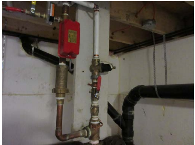
The main water shut off valve is located in the crawl space of the house.
