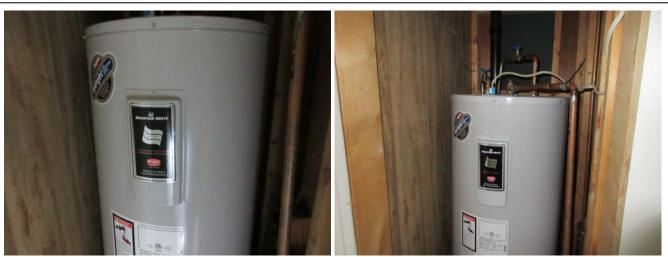
The hot water tank was manufactured dated Feb 2013. The water tank life expectancy is 7-12 years. It has no leaks and is functioning well at the time of this home inspection.
