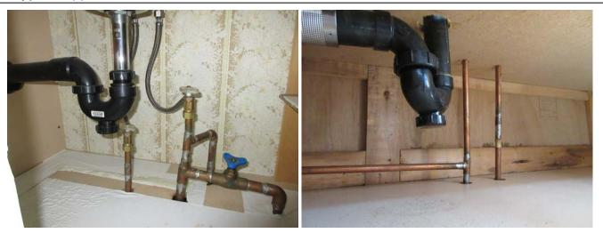
The house original supply pipes is copper. The life expectancy of copper piping is dependent on water condition, it may fail within 20 years. However the copper life expectancy is 40-50 years.
