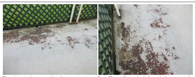
The minor crack was noted on the carport concrete floor. The peeling and missing painting was noted on the concrete slab as well. The crack needs to be monitor for any changes contacting contractor for more action.
