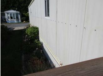
The house has vinyl panel wall cladding and was functional at the time of this home inspection. The wall cladding panel was broken and small portion of the vinyl panel siding damaged. The damaged wall point covered by wood on the north side of the house.
