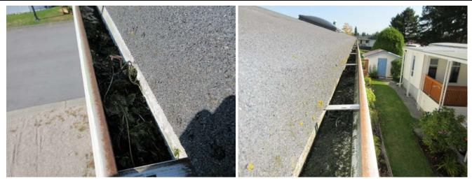
The debris and tree leaves were noted inside of the roof gutter. I recommend clean the gutter to prevent any water leakage to the house.
