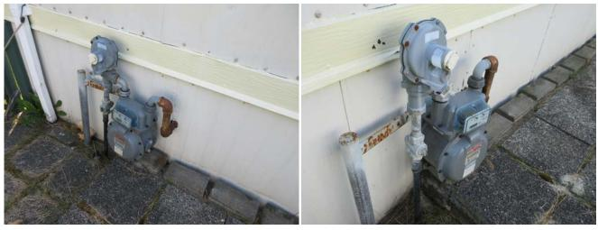
The gas meter was located on the north east of the house. The rust sign was noted on the meter component. I recommend repainting the meter pipe.
