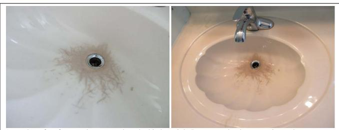
A number of surface crack was noted on the kitchen sink. It seems to be the cosmetic crack.
