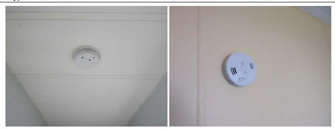
The smoke detector need to be replaced after 10 years and the battery need to be check annually. Replacing smoke detector when moving into a new residence is recommended.
