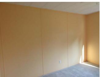
The house had vinyl on gypsum panel. The wall coverage seems to be good and is functioning well at the time of this inspection.
