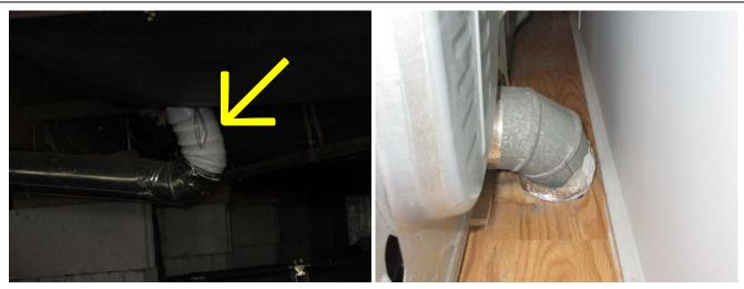
The dryer has small portion of vinyl vent which is not approved for the dryer. The hard metal type vent only is accepted and recommended for dryer. I recommend installing the hard metal duct for the dryer in the laundry room.
