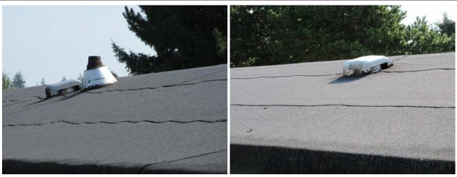
The house roof asphalt rolling coverage. The roof had no leaks and was functioning well at the time of this home inspection.
