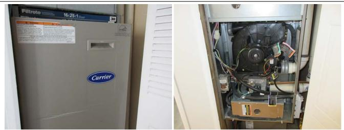
The furnace is a high-efficiency type with input 80000 BTU. The furnace manufactured in dated Apr 2007. The furnace was functional at the time of this inspection.
