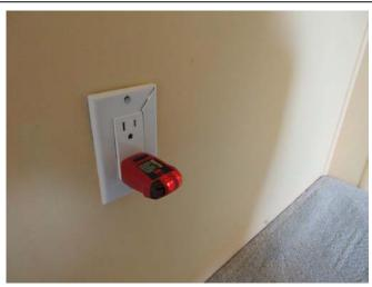
The outlet cover was broken in the master bedroom of the house. I recommend replacing the outlet cover with the new one.
