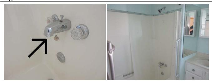
The water leakage was observed on the faucet's spout in the bathroom. I recommend fixing the water leakage.
