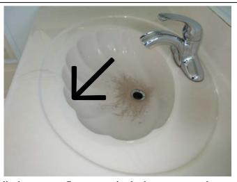
The basin had no hole to discharge overflow water in the basement washroom of the house.
