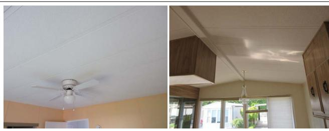
The house ceiling was sheetrock ceilings panel. The ceiling coverage seems to be good and is functioning well at the time of this inspection.
