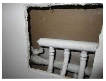
The house original supply pipes is PEX. The life expectancy of PEX piping is 40-50 years. The main water shut off valve is located in the closet of the suite entrance space.
