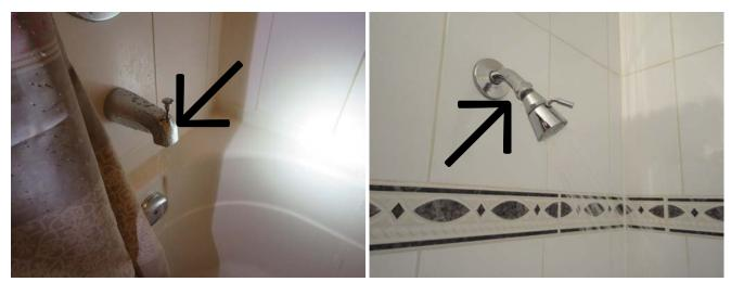
The water leakage was observed on the faucet's spout and shower head at the bathroom. Fixing the water leakage by qualified plumber is recommended.
