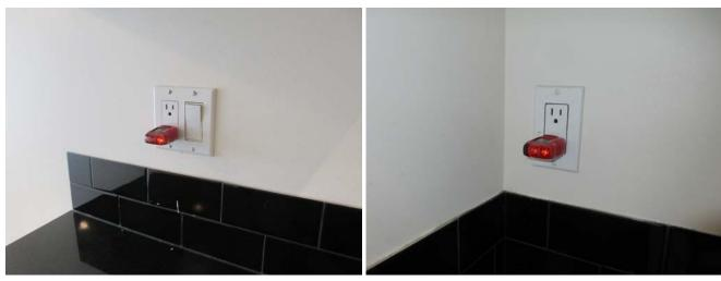
There was no GFCI type outlet in the kitchen. It is safety concern. The outlet needs to be GFCI type in the kitchen to protect users from any electrical shock and unsafe situation. Ground Fault Circuit Interrupter (GFCI) outlets are recommended for installation at kitchen outlets.
