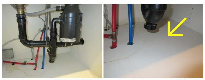
The water leakage was noted under the kitchen sink sewage pipe of the house. I recommend fixing the water leakage.
