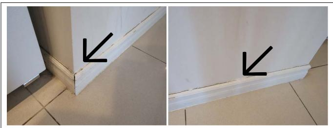
The wood baseboard had cracks and was separated in the kitchen and entrance space of the house. Repairing the wood baseboard is recommended.
