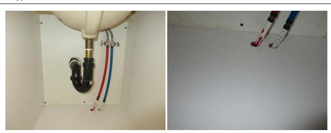
The water leakage was noted under the basin faucet. I recommend fixing the water leakage.
