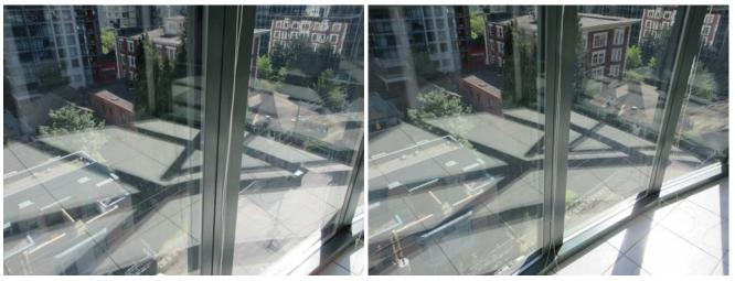
The sealant of the window glass was broken in the study room of the house. The condensation was noted inside the double pane. Fixing the window pan to prevent heating lose is recommended.
